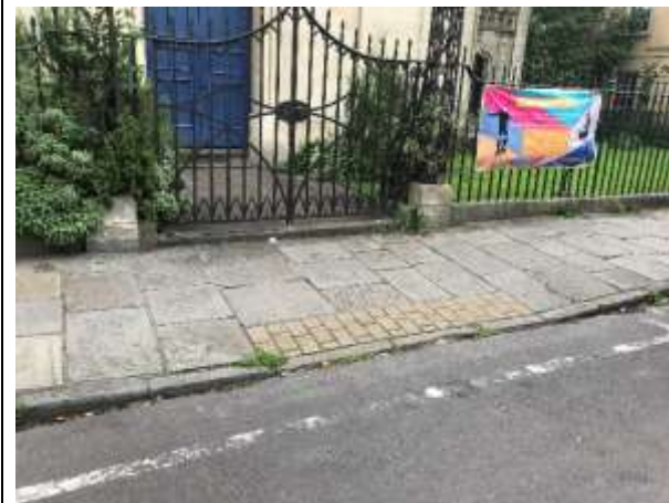
Dropped kerb outside Circomedia.
