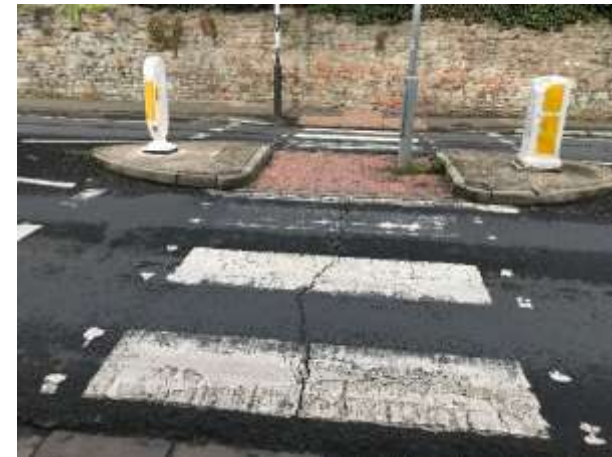
Zebra crossing on City Road, pedestrian refuge point and tactile indicators and dropped kerbs.
