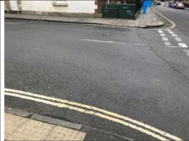
Wilson Street crossing point, dropped kerbs, tactile indicators and uneven paving
